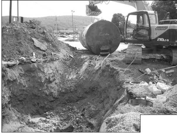
Figure 1.8 Excavation of a leaking 30 kL steel tank from a former retail petroleum site. Photo courtesy of Joshua Gowan.
